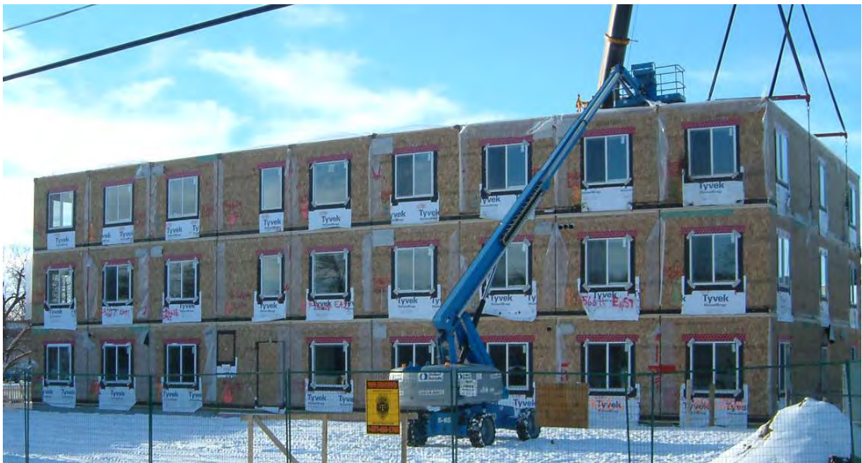
Figure 29: Canora Place: 27 Modules Set at -32 Degrees Celcius
