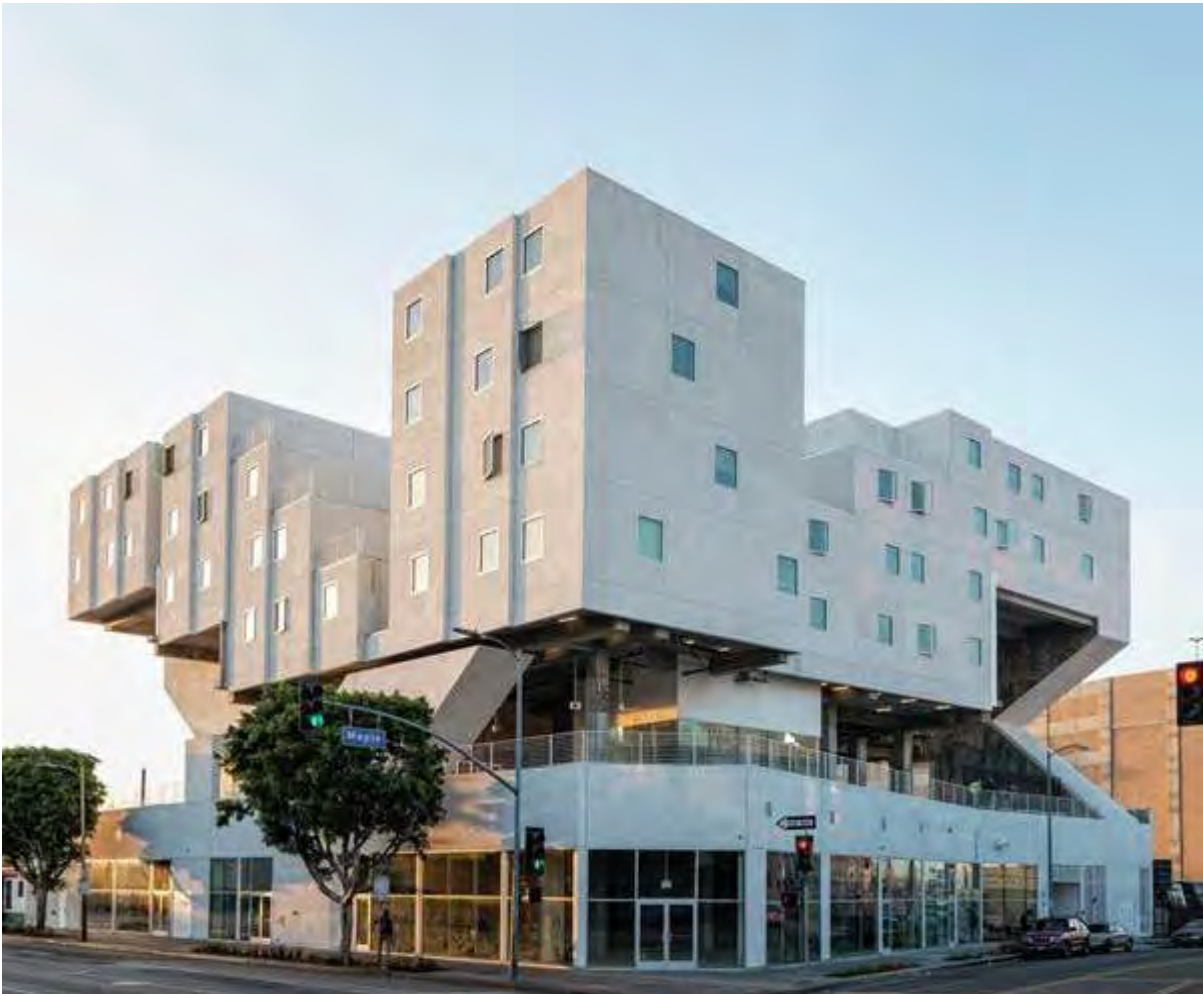
LA's Star Apartments: modular and prefabricated, six-storey residence built for Skid Row Housing Trust, LEED Platinum pending. Photo used with permission from Gabor Ekecs.
