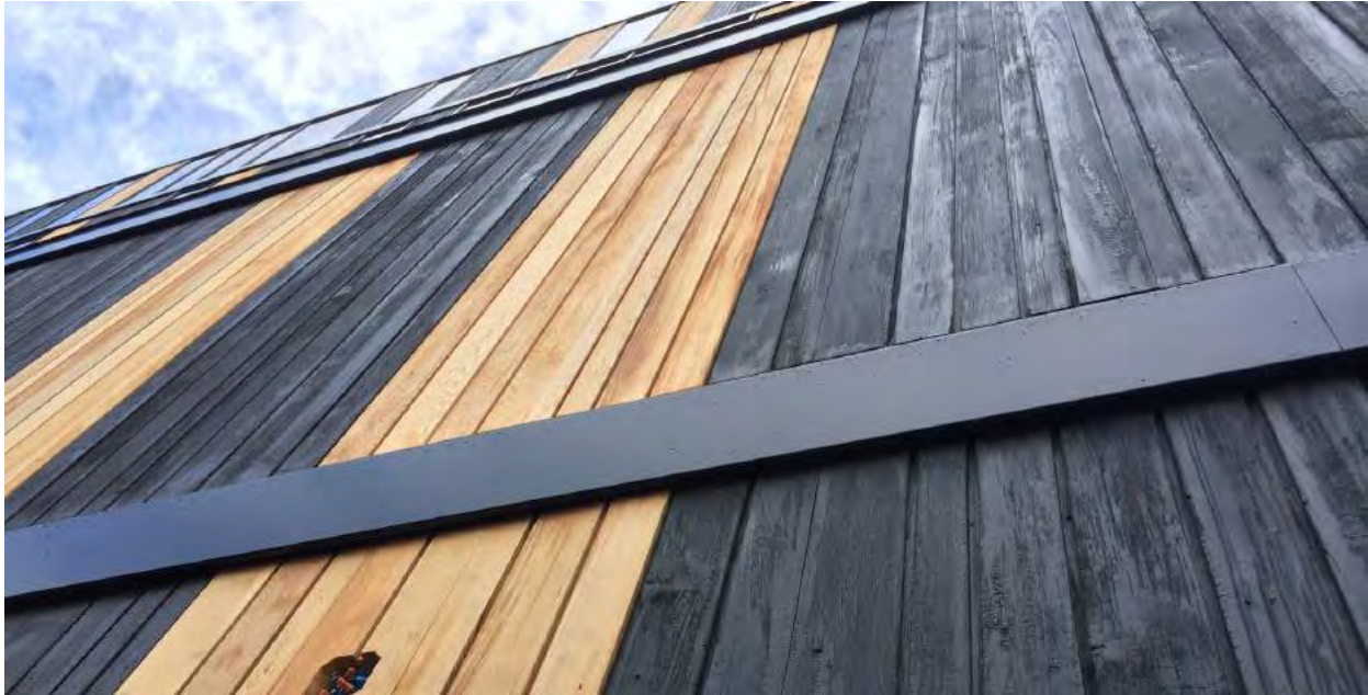
Figure 9: Exterior Char Layer, Wood Innovation and Design Centre, Prince George
