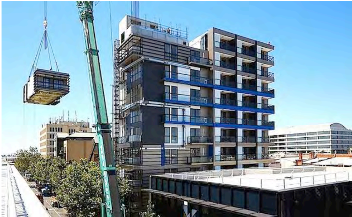
Figure 13: One9 - Nine storey, Steel Frame Melbourne Apartment Built in Five Days
