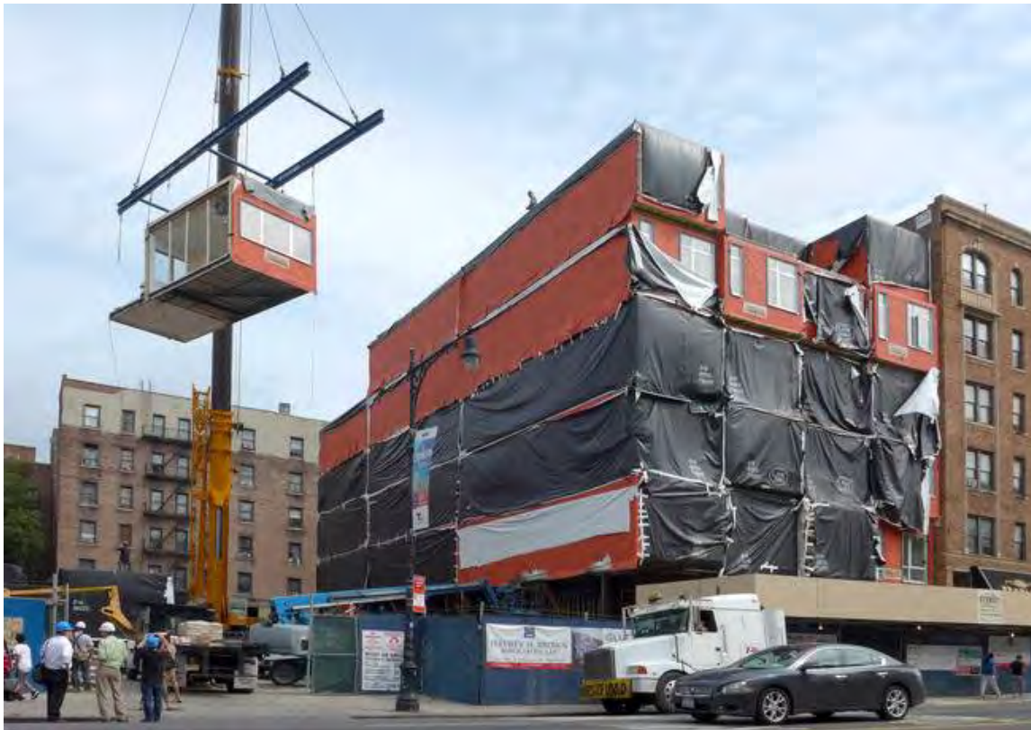
Figure 15: The Stack: NY's Tallest Modular Project is Steel Framed
