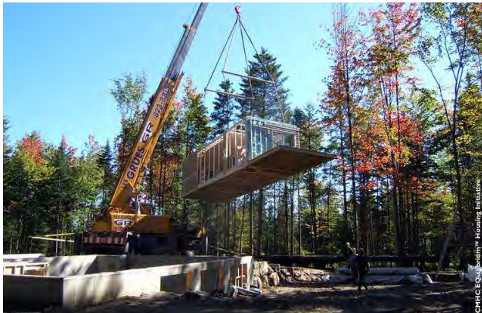
Figure 18: First ÉcoTerra™ Module Installed on Poured-In-Place Basement
