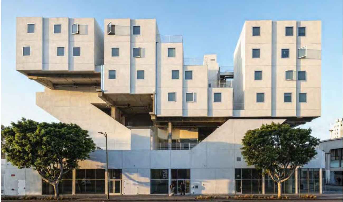
Figure 30: LA's LEED Platinum Star Apartments: 6 Storey Modular Residence
